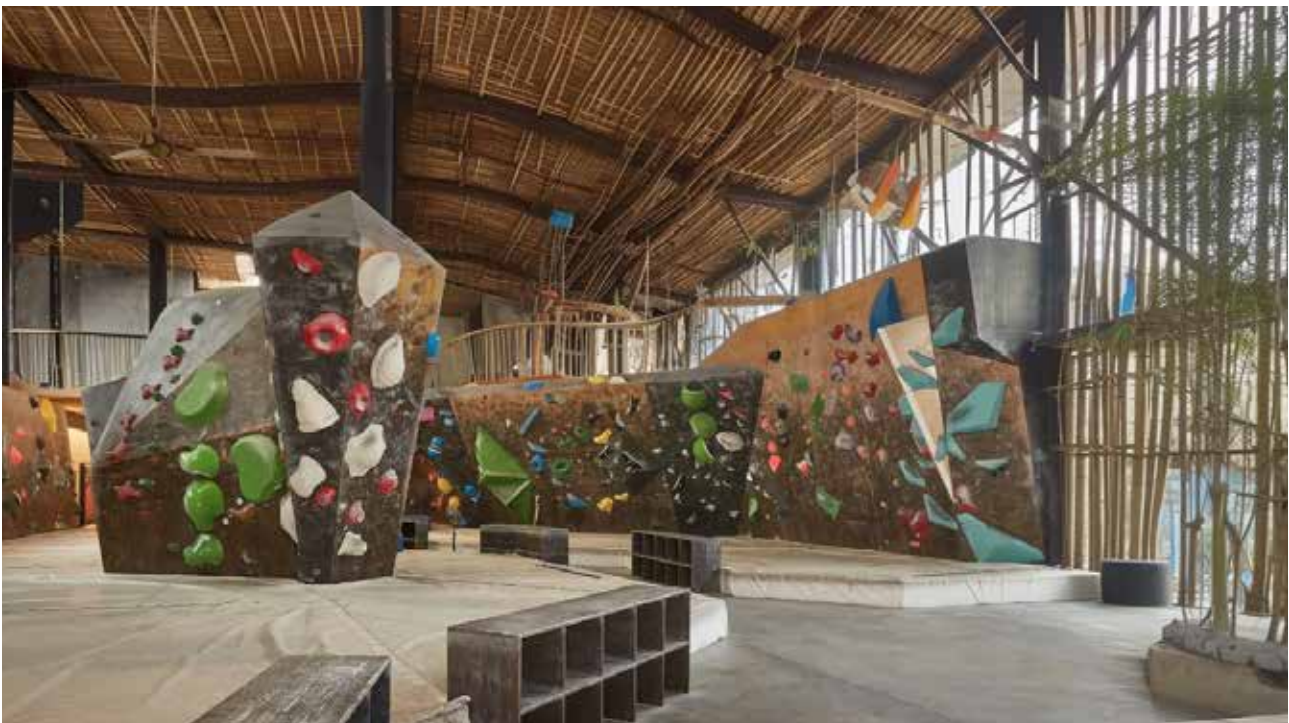
The bouldering hall consists of a shell made of local sustainable materials and climbing wall elements made of multi-layered maritime pine panels.
